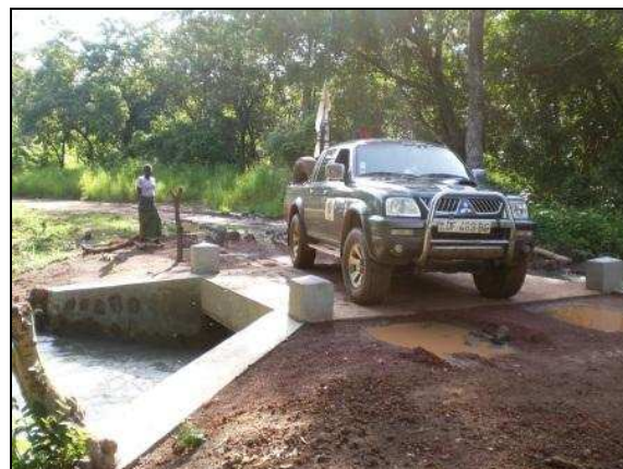
...and after the rehabilitation of the Yambala bridge
